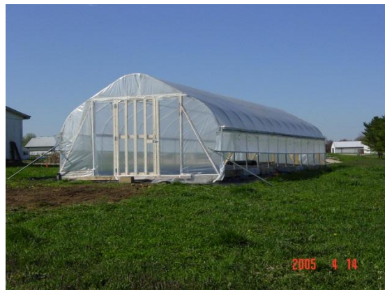
Figure 4. SARE project coordinator Bryan Butler helped build this high tunnel, illustrating a useful end wall with a large door, on a University of Maryland research farm.
