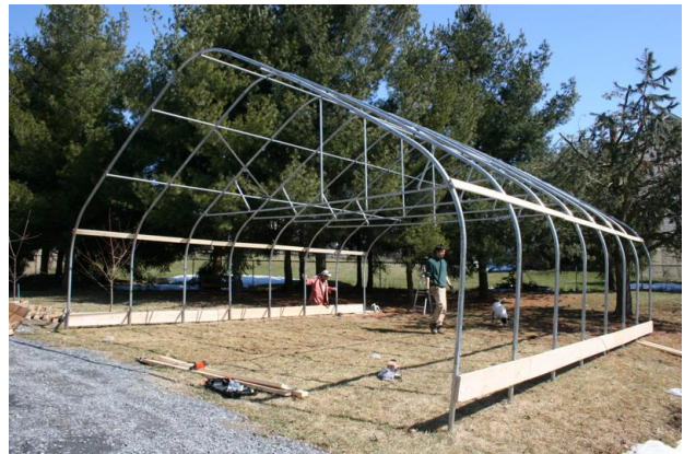
Figure 3. The skeleton of this tunnel, built between a driveway and a grove of trees, illustrates that growers need not have a perfect site for the structure. This tunnel was customized to maximize the available space.
