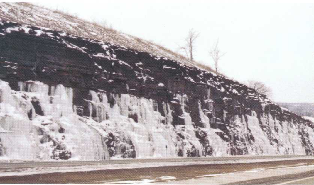
Ground water, emerging from bedding planes, has created spectacular frozen waterfalls along a road cut.
