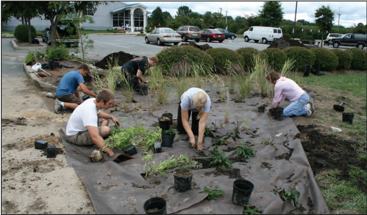
Figure 31. Lower Eastern Shore Tributary Team members and volunteers planted native grasses, flowers, and shrubs at one of two rain gardens installed at the Providence Presbyterian Church in Salisbury, MD.
