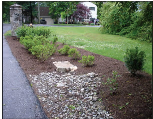
Figure 5. The rain garden installed across from the Highland Beach Town Hall drains water after each storm. Well designed rain gardens drain 24-48 hours after a storm.
