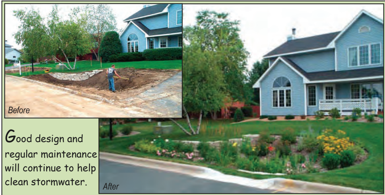
Figure 34. A Burnsville, MN home before and after rain garden construction. The City of Burnsville, MN constructed rain gardens to improve the water quality of Crystal Lake by adding rain gardens to a 20-year-old neighborhood. To learn more about the project visit http://www.landandwater.com/features/vol48no5/vol48no5_2.html .
