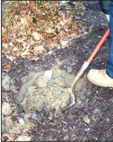
Figure 38. Dig a hole first.
