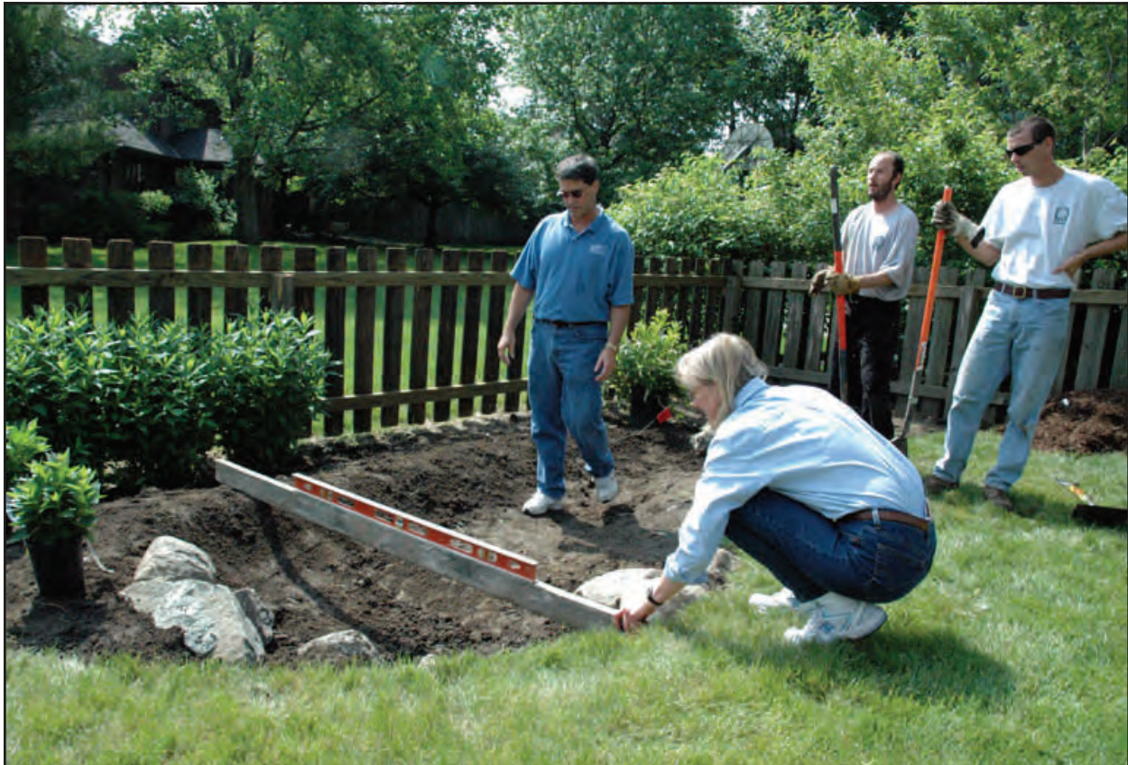
Figure 25. If your level is long enough, use it to level the height of your rain garden berm.
