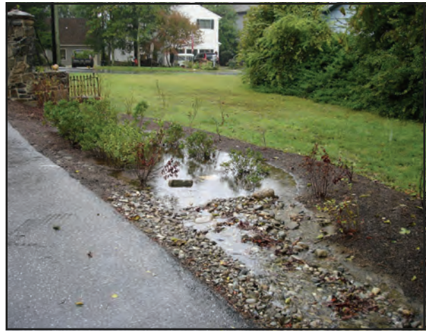
Figure 4. Don't be surprised if your rain garden has water in it after a storm. It's supposed to. The rain garden installed across from the town hall in Highland Beach, Maryland is strategically placed to collect runoff from the road and lawns.
