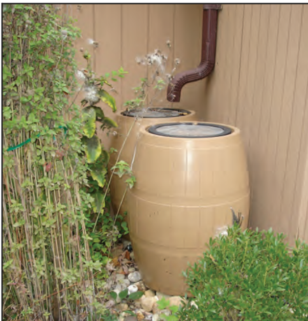
Figure 37. Connected rain barrels at Arlington Echo.
