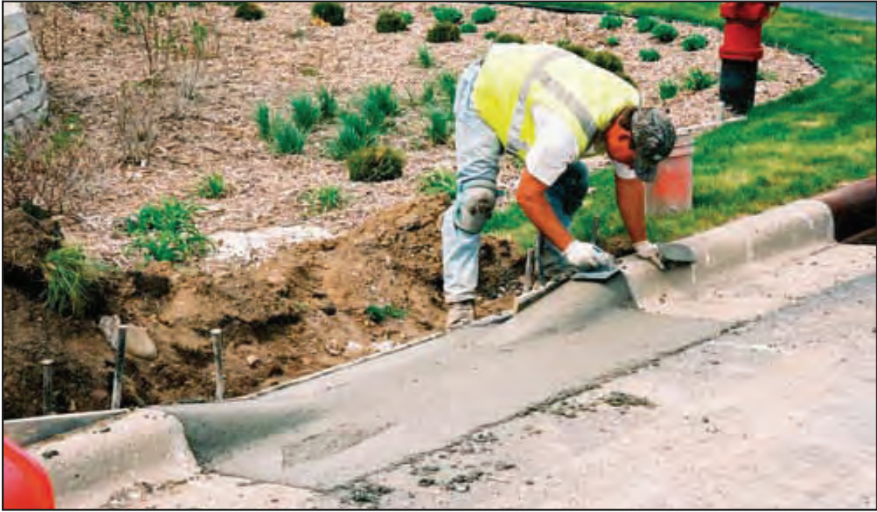
Figure 21. Creating a curb cut allows stormwater runoff from streets to enter rain gardens.
