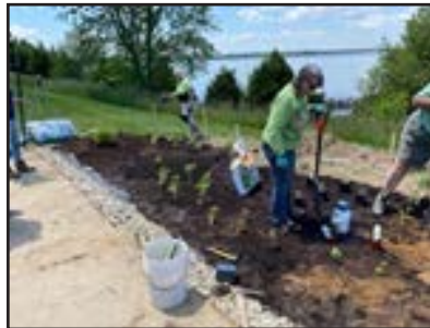
◀ Stewards prepared the site, amended the soil to allow for infiltration and planted the garden with 7 different varieties of native perennials that will add to the aesthetics of the area.
