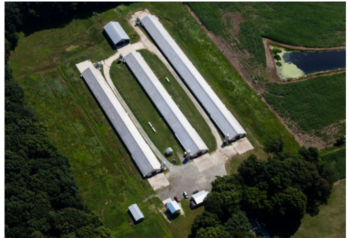
Poultry barns in Maryland. Image by Chesapeake Bay Program
