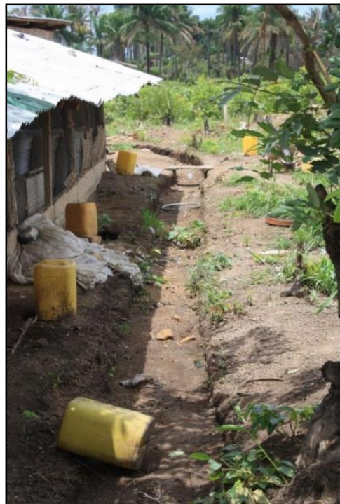
Good storm water drainage
