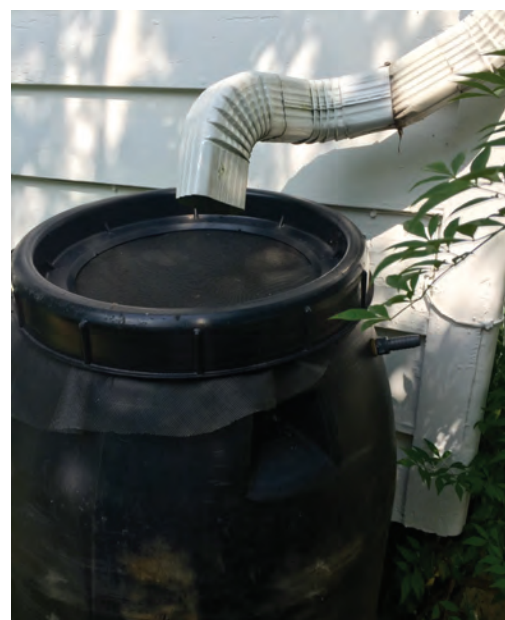
Figure 5.10. Rain Barrel with open top, 2 layers of screen, and downspout entering above. This allows for some pre-screening of leaves and debris as well as a strategy to prevent mosquitoes from entering.
